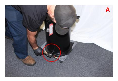
TO SEPARATE THE LID AND PICK UP TUBE ASSEMBLY FROM BARREL THERE ARE TWO OPTIONS.
